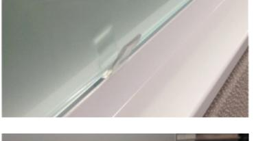
STEP 16: Installation of privacy glass is complete with shiny side out and logo on the bottom left corner
